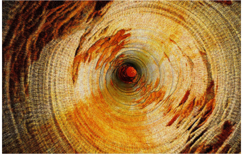
Stress-induced damage can be easily identified in Hovermap data. Buckling and stress-induced spalling perpendicular to the principal stress direction can be observed in this vent raise.
